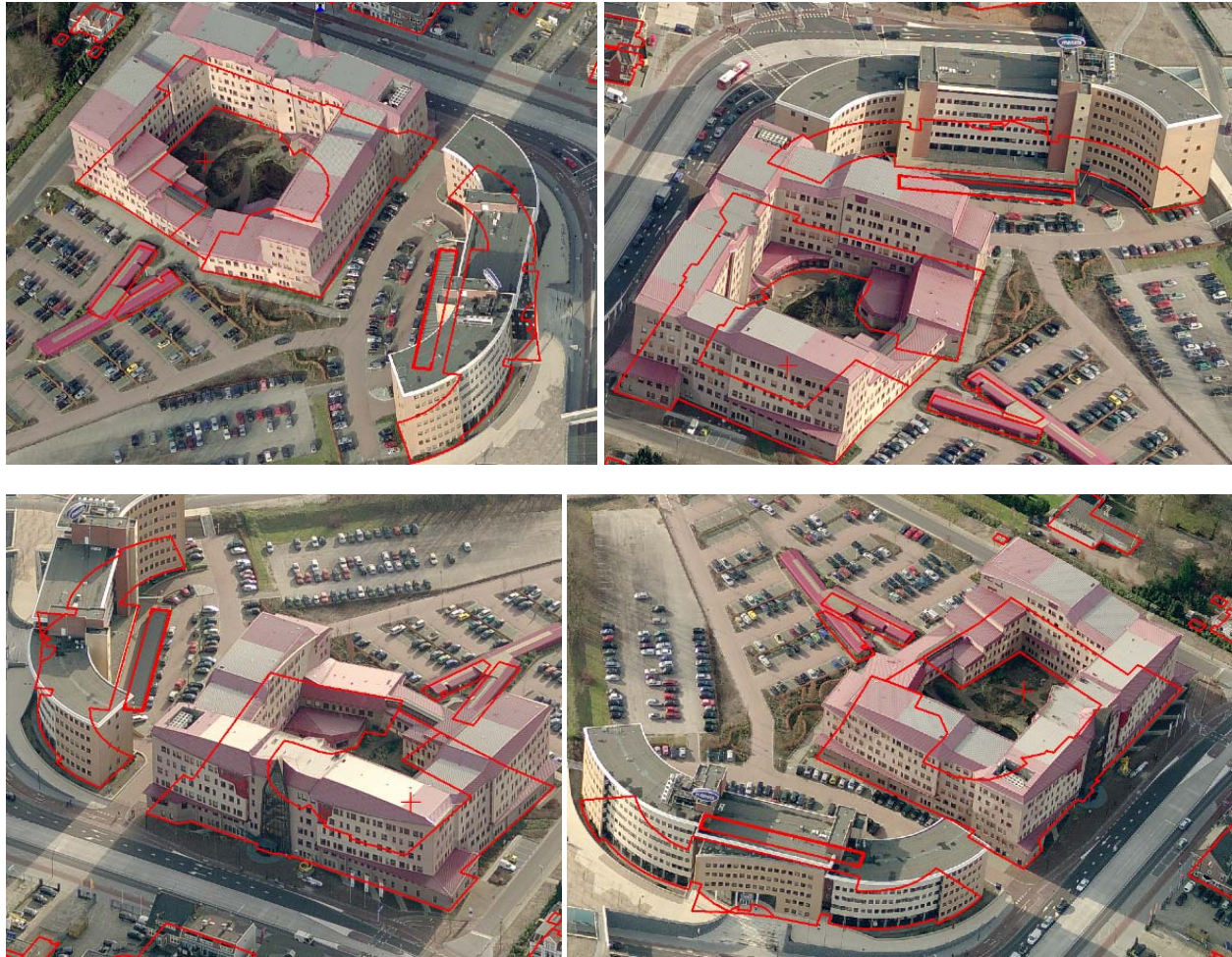
Figure 1. Different oblique views of buildings overlaid with 2D GIS data. Images:©Blom
