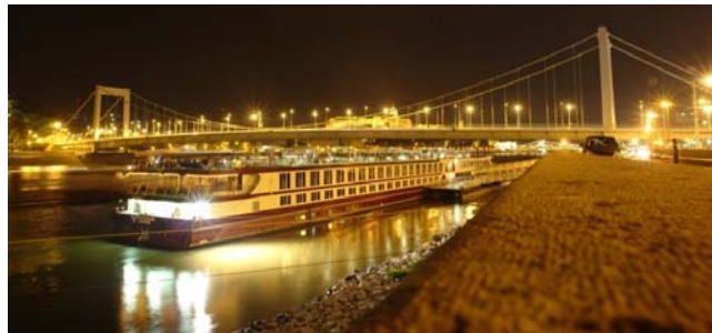
Figure 10. Erzsébet Bridge from the first scanning station.
