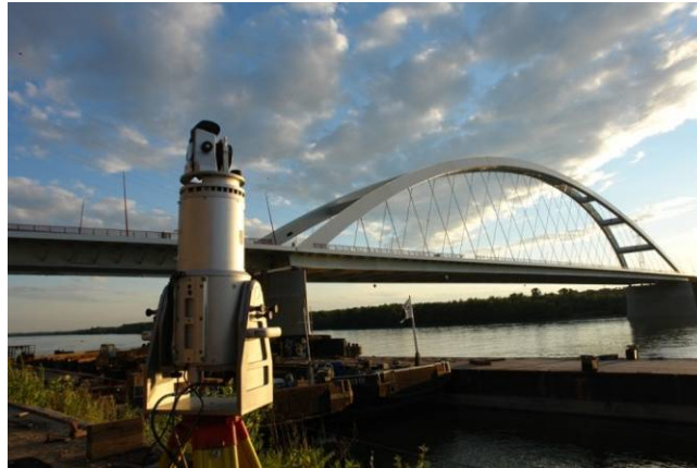
Figure 1. Laser scanning the Pentele Bridge.
