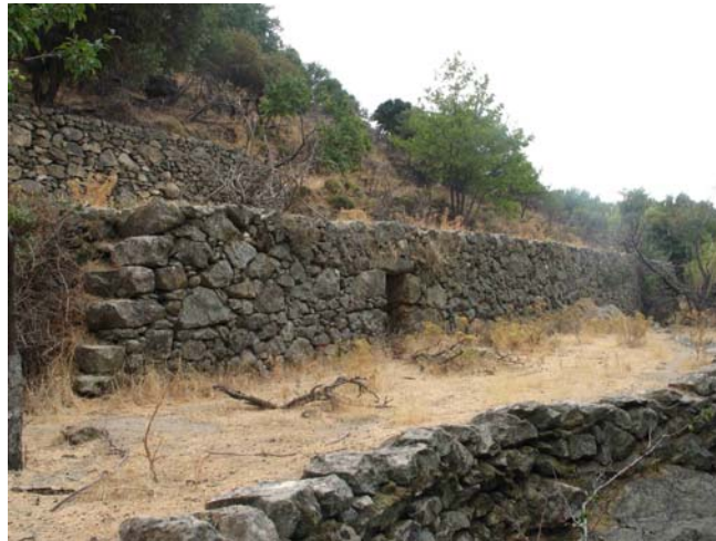
Figure 6. Detail showing abandoned agriculture with terraces. In the middle is showing a small opening in the wall to protect people from the rain.
