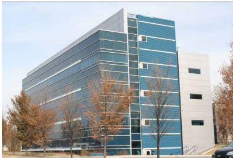
Figure 2. “CCIT” building, University of Calgary, Canada.
