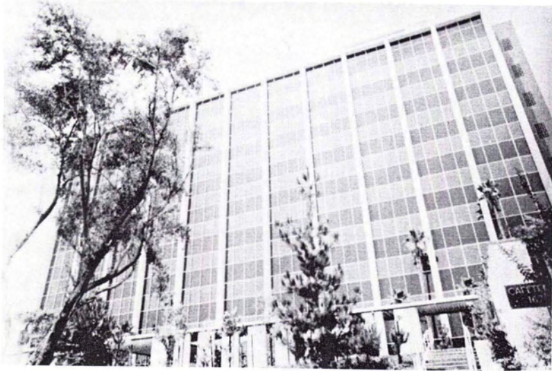
FIG. 9. Building distorted by camera lens, prior to perspective rectification (courtesy of Jet Propulsion Laboratory/Image Processing Laboratory).
