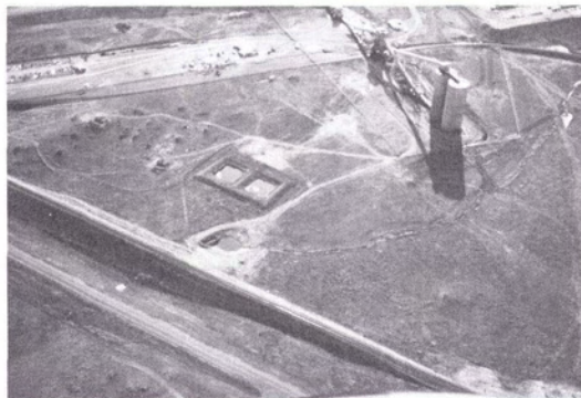
FIG. 2. Low oblique aerial photograph.
