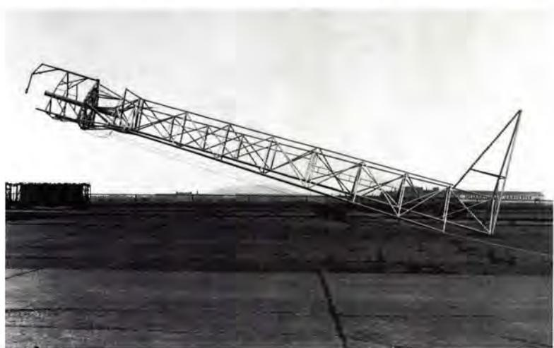
Figures 4 and 5. Park's survey observation-tower units, at left in the upright position; above, the tower is being lowered.
