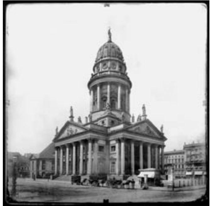
Figure 2. The French Cathedral in Berlin, a photograph taken by Meydenbauer in 1882. 100 years later the image was used for reconstruction purposes because the church was heavily damaged in World War II.
